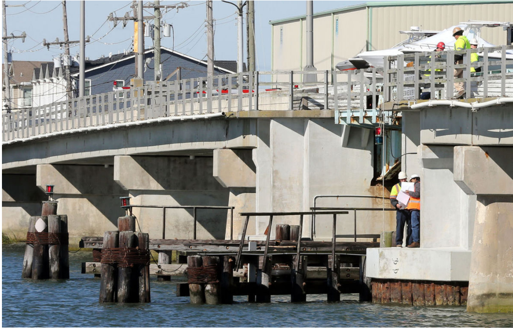
96 th Street Bridge
